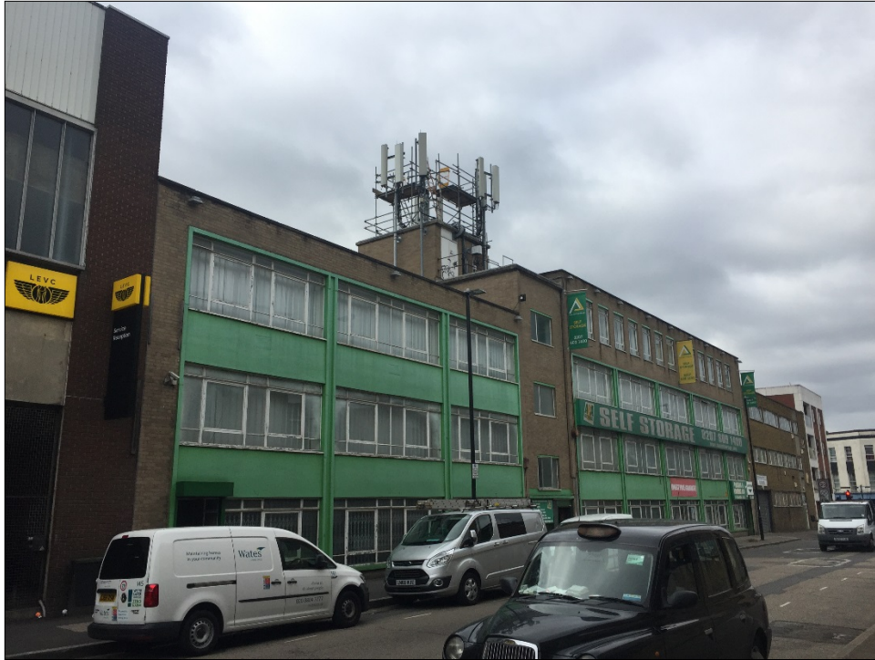
Photograph 4: Brewery Road elevation, looking west.
