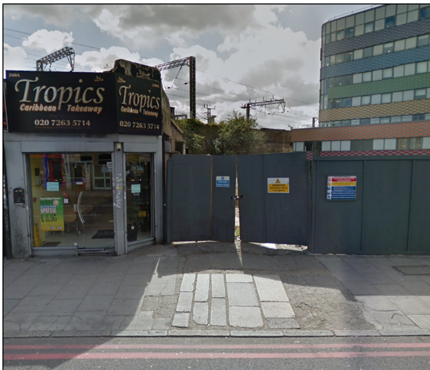
Figure 3: Photo showing pre-existing crossover and vehicular entrance into 240 Seven Sisters Road.
