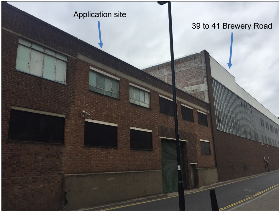
Photograph 6: Brandon Road elevation looking east.
